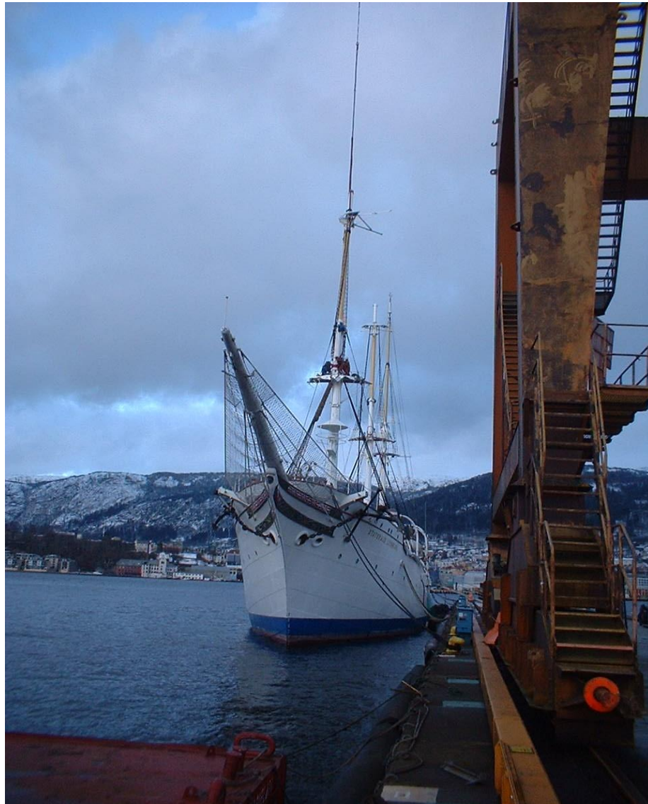
Installing overhauled fore topmast
